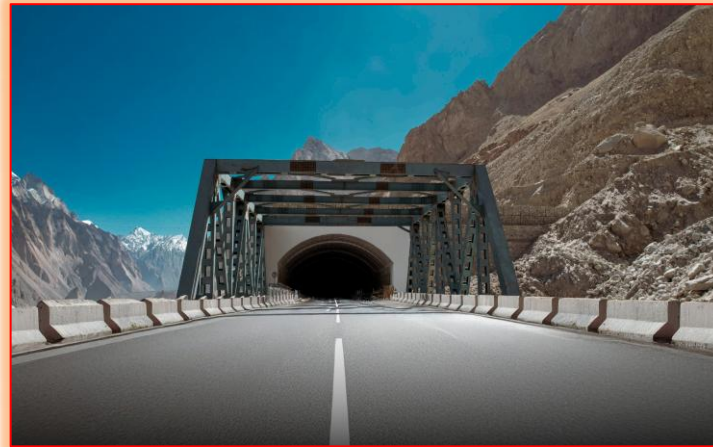
Precast Cut-and-Cover Tunnel, Leh, Ladakh
