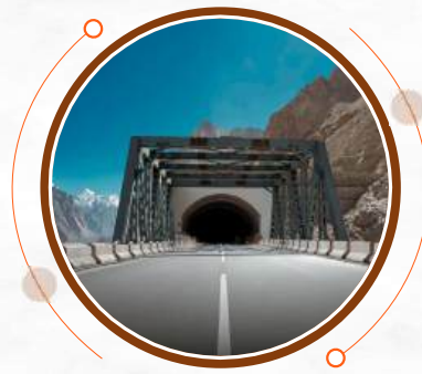
Precast Cut-and-Cover Tunnel, Leh, Ladakh India's Longest Precast Cut-and-Cover Tunnel – Leh, Ladakh
