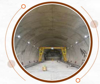
Cavern, Hanle, Ladakh, BRO India's Highest Underground Cavern – Hanle, Ladakh
