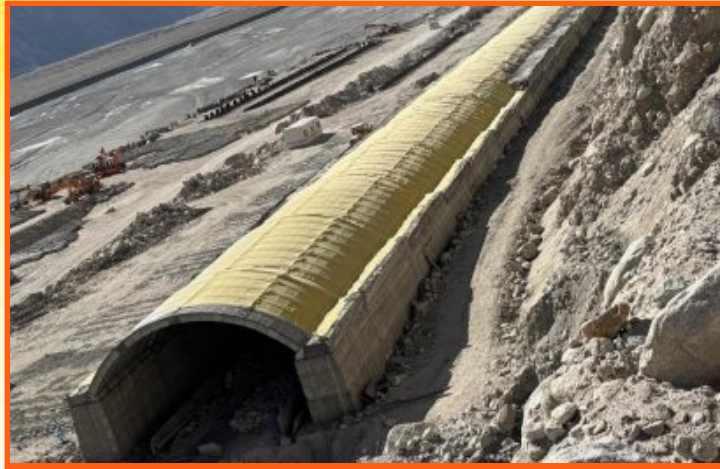
Precast Cut-and-Cover Tunnel, Leh, Ladakh
