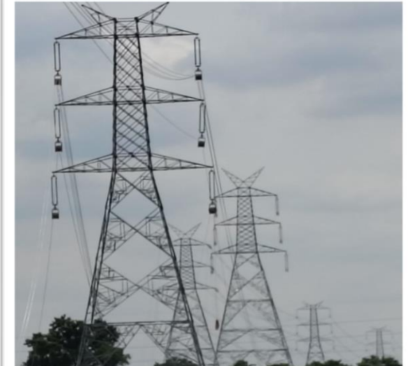
400kV DC Koppal to Gadag Transmission Line Project
