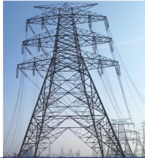
TNEB 400 kV DC MC Transmission Line Project.
