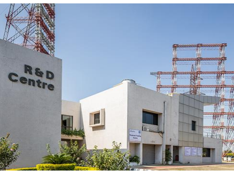
Tower Testing Facility - Deoli
