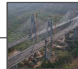
The Mumbai-Pune Missing Link India's tallest road cable-stayed bridge at Mumbai-Pune Expressway
