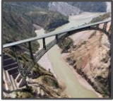
Chenab Bridge World's tallest single-arch railway bridge
