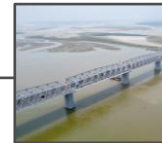
MG Setu 1 st time in India – replaced existing concrete superstructure with new steel superstructure
