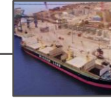
New Owendo International Port, Gabon Fastest completion of port project in West Africa
