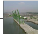
JNPT, Mumbai India's largest container port; Constructed 1 suspended deck wharf and 5 approach trestles
