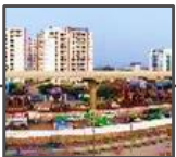
Kanpur Metro Constructed in record time of less than 2 years despite the Covid-19 pandemic
