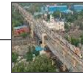
Nagpur Metro India's 1 st 4-layer transportation system at Gaddigodam Railway Crossing
