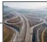
Package 14, Igatpuri India's widest and Maharashtra's longest road tunnel at Nagpur Mumbai Expressway
