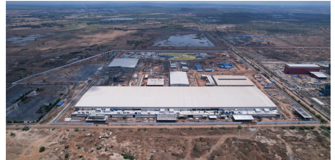
External view of upcoming cell plant at Naidupeta
