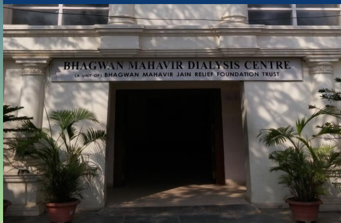
Installed 60 kW rooftop solar plant at Bhagwan Mahavir Dialysis Centre, supporting clean energy for healthcare
