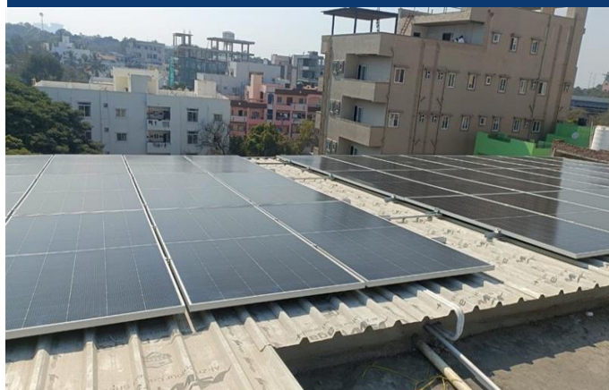
Commissioned 50 kW rooftop solar plant at Thalassemia Sickle Cell Care Centre to support clean energy for healthcare
