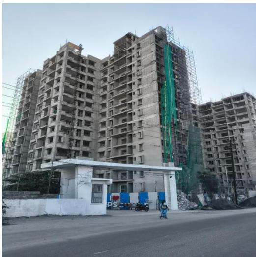
TULIPS PHASE 3, BUILDING 7 COIMBATORE
