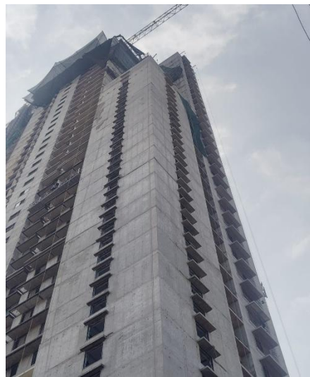
MUMBAI METRO HIGH-RISE BUILDING
