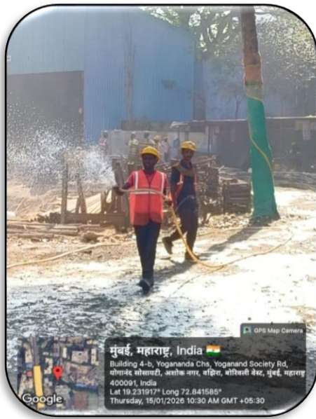
Water spraying for dust suppression
