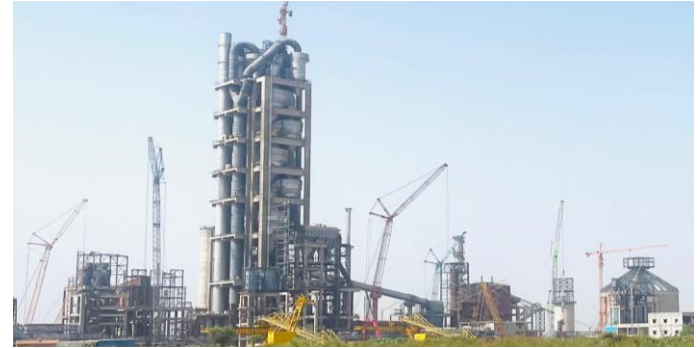
Nagaur IU – pyro processing and clinker silo
