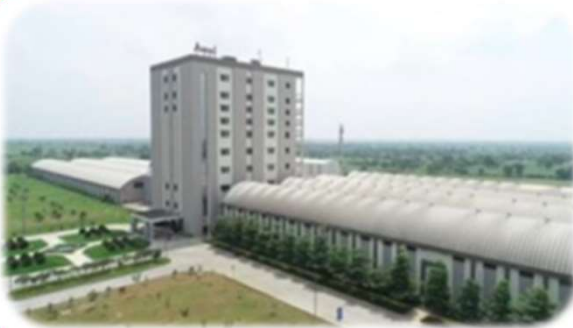
Self-supported roofing structure for a major Indian milk co-operative society at Anand Gujarat
