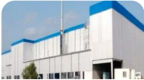
Over 62,000 sq. m. PEB installation for the automobile manufacturing plant of a global automobile manufacturer located at Ahmedabad, Gujarat
