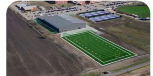
Over 5,500 sq. m. PEB installation for an indoor multi-use facility at Texas, US
