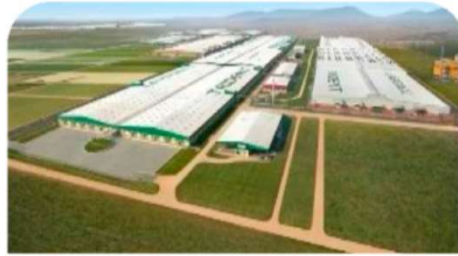
Over 285,000 sq. m. PEB installation for a textile plant for a major textile company at Hoshangabad, Madhya Pradesh
