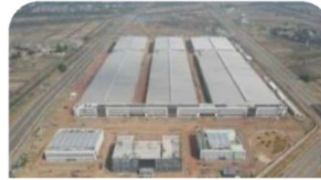
Over 125,000 sq. m. PEB installation for a multinational home appliance manufacturer based out of Noida
