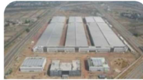
Over 125,000 sq. m. PEB installation for a multinational home appliance manufacturer based out of Noida
