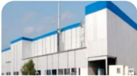
Over 62,000 sq. m. PEB installation for the automobile manufacturing plant of a global automobile manufacturer located at Ahmedabad, Gujarat
