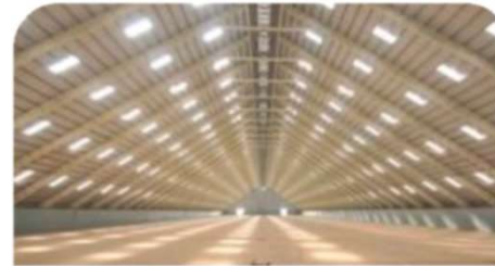
Approx 90,000 sq. m. 'A' frame structure with a centre height of 42 metres and clean span of 84 metres specially designed for the sugar storage requirements for a major Indian sugar company in Kandla, Gujarat
