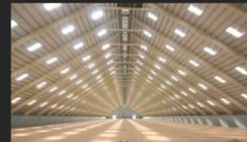
Approx 90,000 sq. m. 'A' frame structure with a centre height of 42 metres and clear span of 84 metres specially designed for the sugar storage requirements for a major Indian sugar company in Kandla, Gujarat
