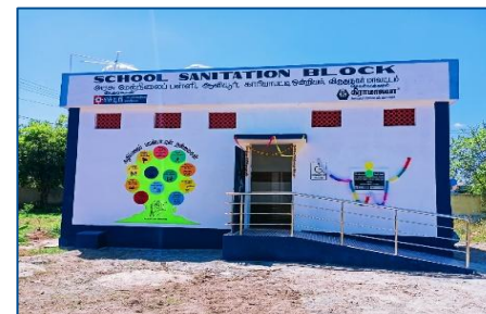
Safe Sanitation Complex, WASH
