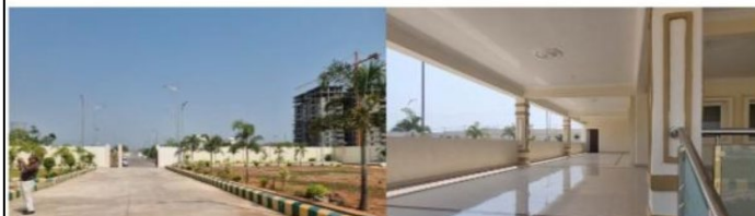
Integrated Township, Nalgonda, Telangana
