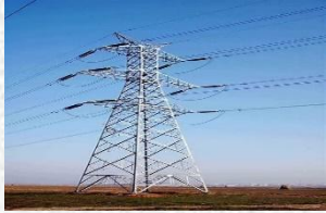
Power Transmission Tower
