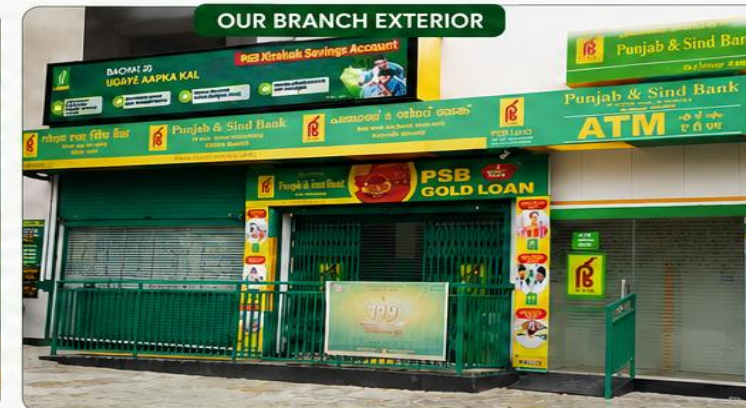
OUR BRANCH EXTERIOR
