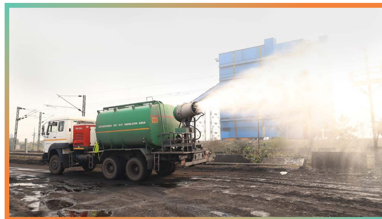
► Fog Cannon for effective dust suppression
