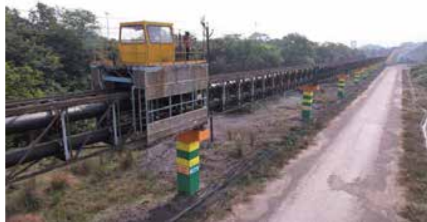
► Eco-sensitive 5 Km Pipe Conveyor at Lakhanpur
