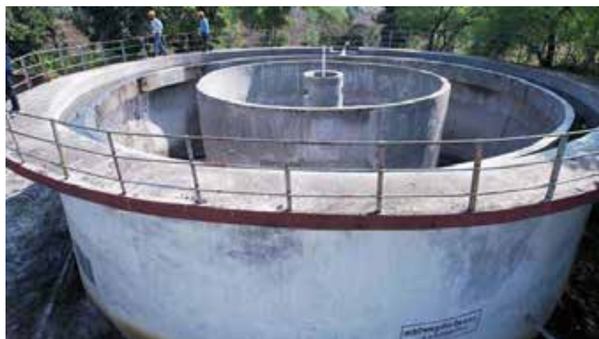
► Khairaha Sohagpur Mine Water Treatment plant
