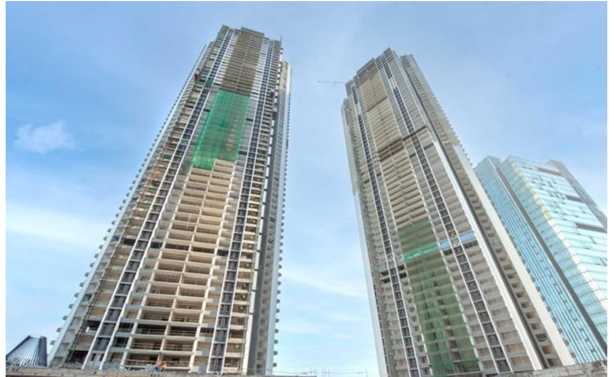
Tower – A & B
