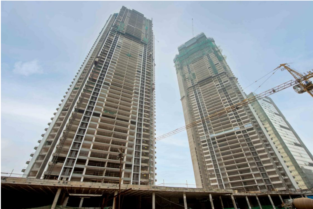
Tower – A & B
