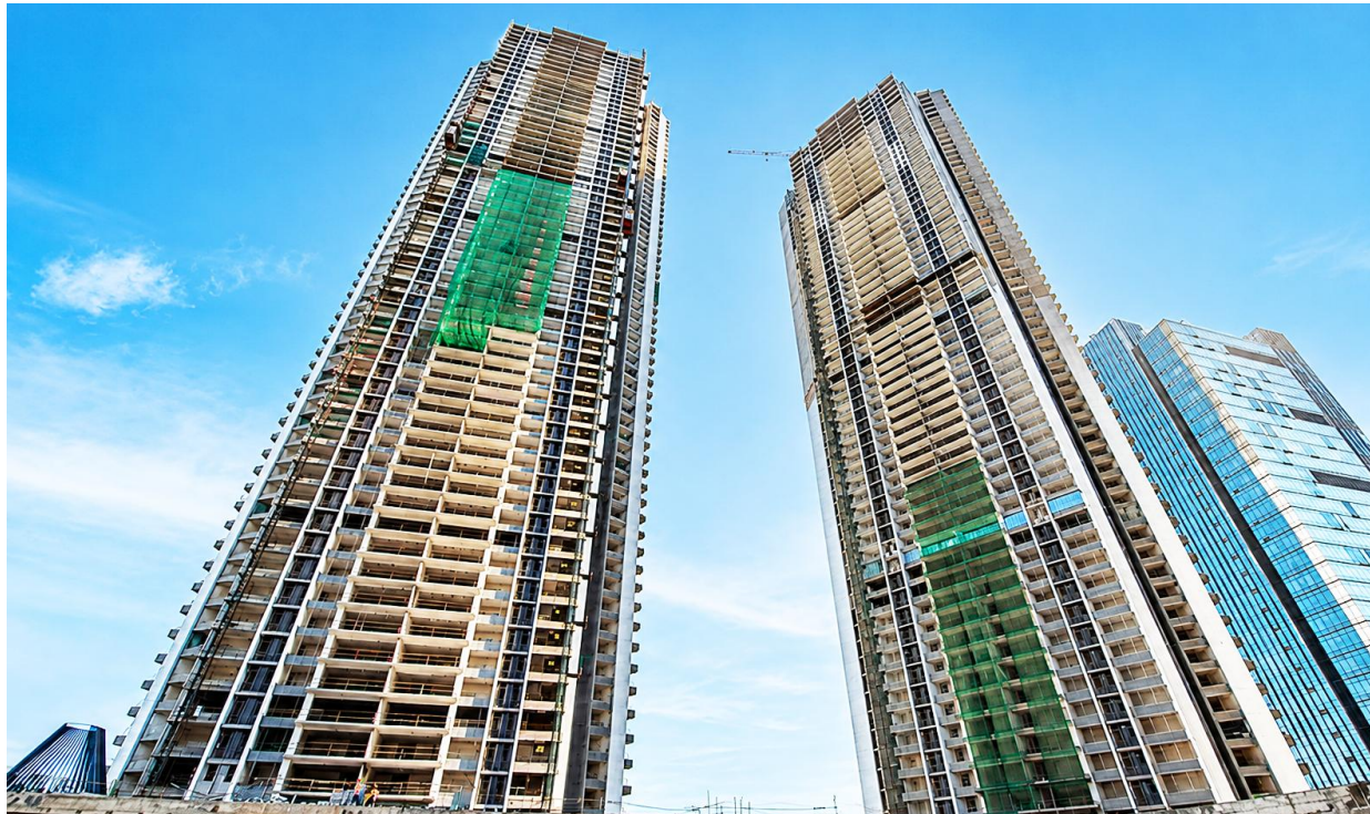
Towers – A & B
