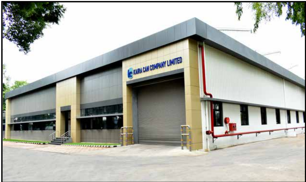
Kanjari Factory - Gujarat
