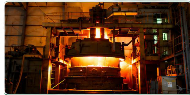
Two Ladle Refining Furnace
