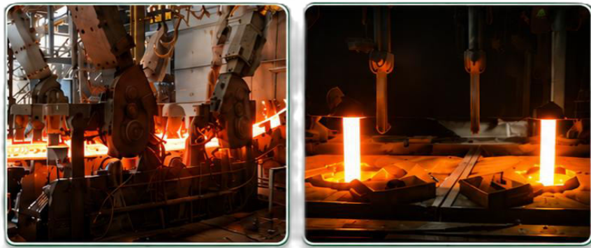
Continuous Casting Machine
