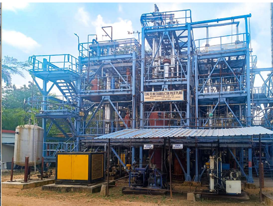
1.2 TPD Coal Gasification pilot plant for producing 0.25 TPD Methanol from high-ash coal established by BHEL at Hyderabad
