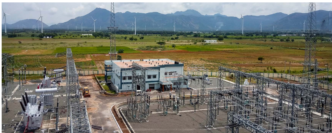
400/ 110 kV TANTRANSCO Thappagundu air insulated substation executed by BHEL in Tamil Nadu
