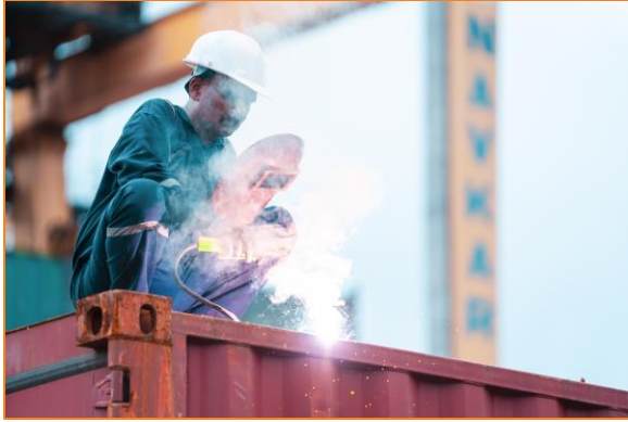
Container's repair and maintenance
