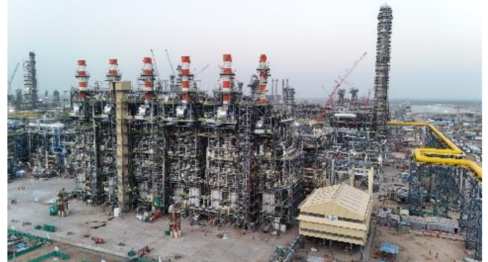
HRRL Project, Rajasthan
