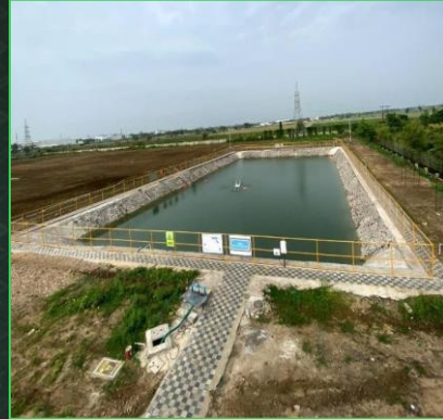
Rainwater Harvesting pond
