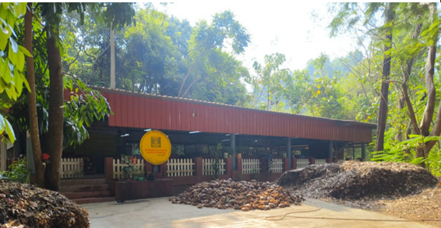
Sustainable Waste Management: MRPL's In-House Vermicomposting Initiative
