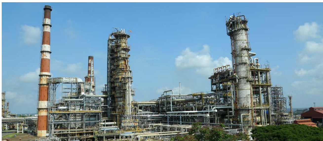
Crude Distillation Unit - Phase 2
