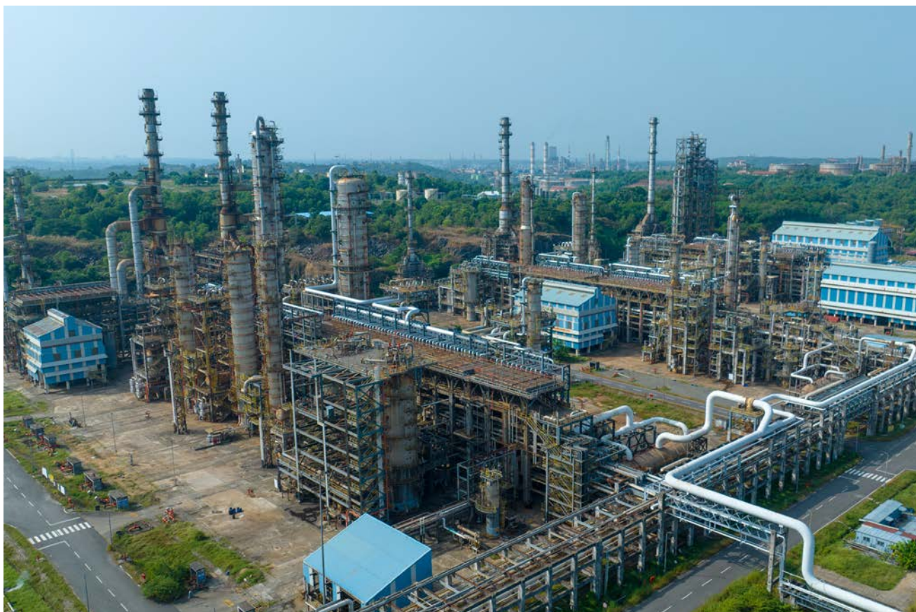
Aromatic Complex, Block-2 Process Units
