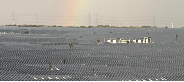
2012 MWp Ground Mounted project at Bikaner, Rajasthan
