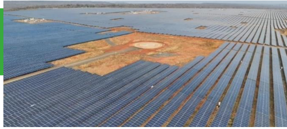
980 MWp Ground Mounted project at Kurnool, Andhra Pradesh
