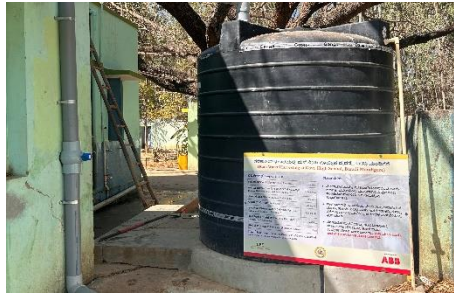
Rainwater harvesting and storage for use as part of Green Campus program
