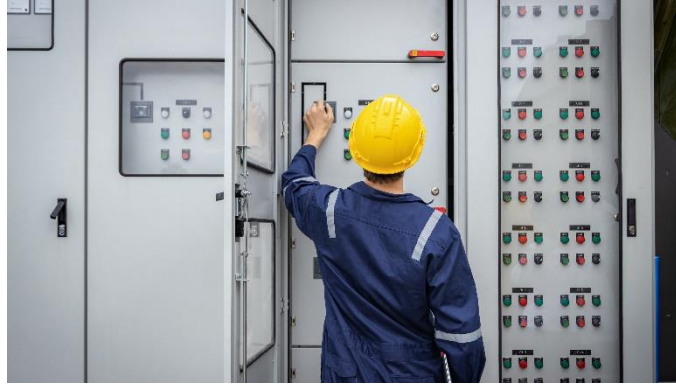
Air Insulated Switchgear panels for a petrochemical company
