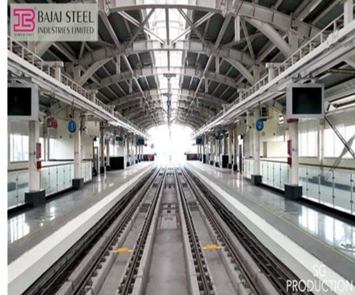
Metro Station, Nagpur – Fire Fighting System
