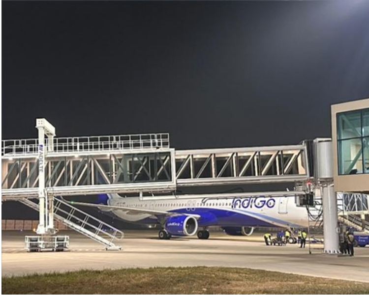
Passenger Boarding Bridge
