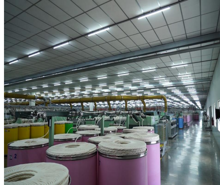
Electrification work of Spinning Mills
