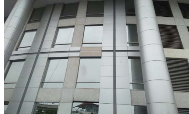
Fibre Cement Boards DLF Cyber city, Gurgaon
