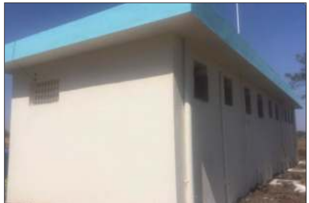
Construction of toilets for girls
