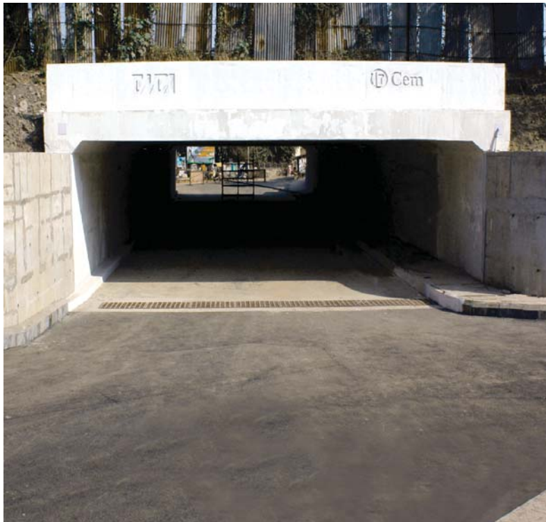
Box Pushing below Rail Track, Kolkata
