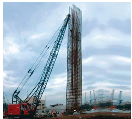
Construction of Diaphragm wall, Delhi
