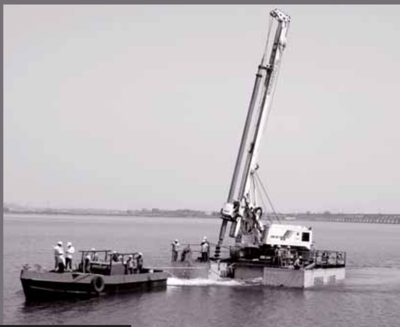
Piling Work, Cuttack, Odisha
