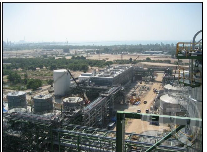
Piping works for PTT phenol project
