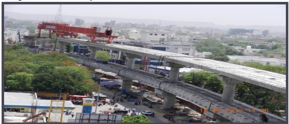
Jaipur Metro Rail Project
