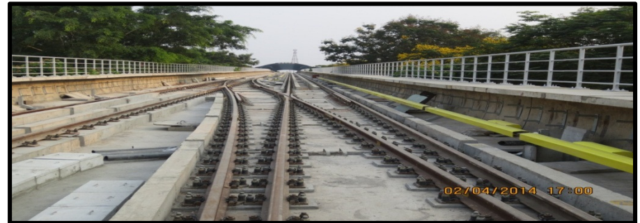
Bangalore Metro Rail Project
