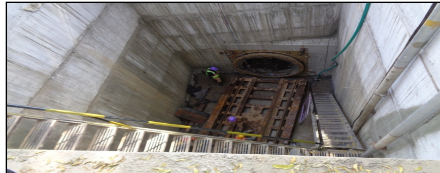
VMSS – Micro Tunneling Vadodara
