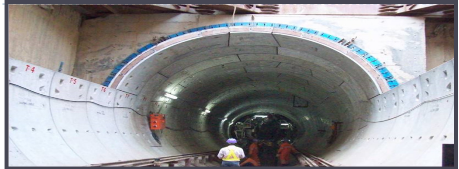
Tunnel work for DMRC
