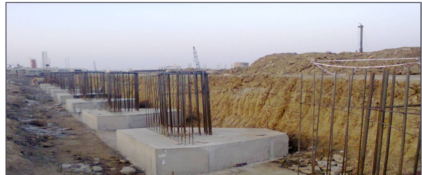
Foundation BASF, Dahej
