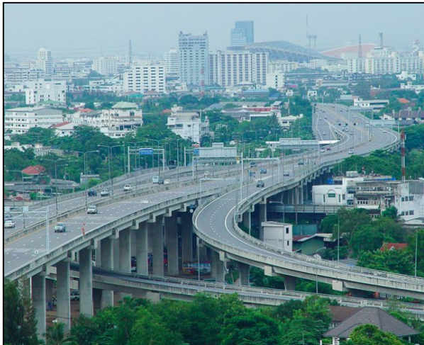
Ramindra - At Narong Expressway System
