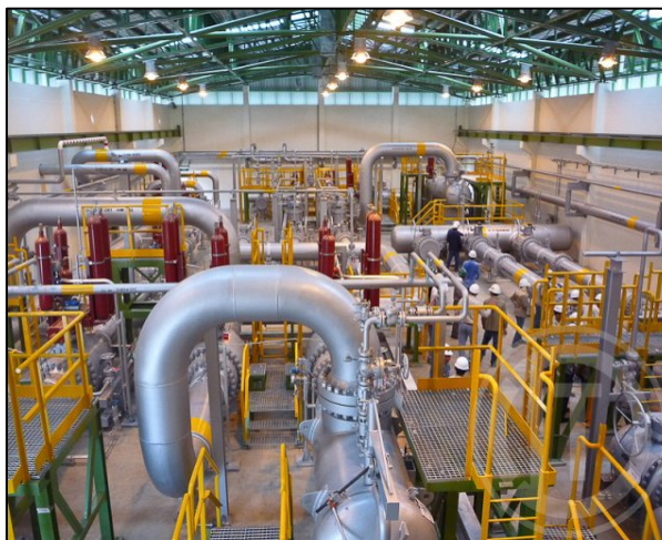
North Bangkok Power Plant Gas Pipeline Project
