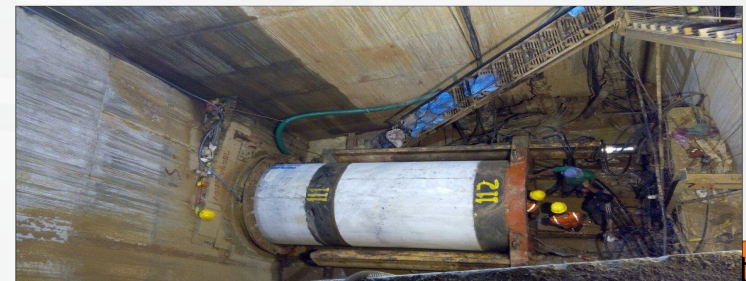
VMSS – Micro Tunneling Vadodara
