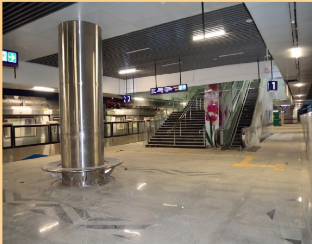
Delhi Metro Palam Underground Station
