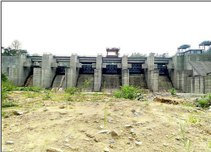
New Hydro Dam Umtru
