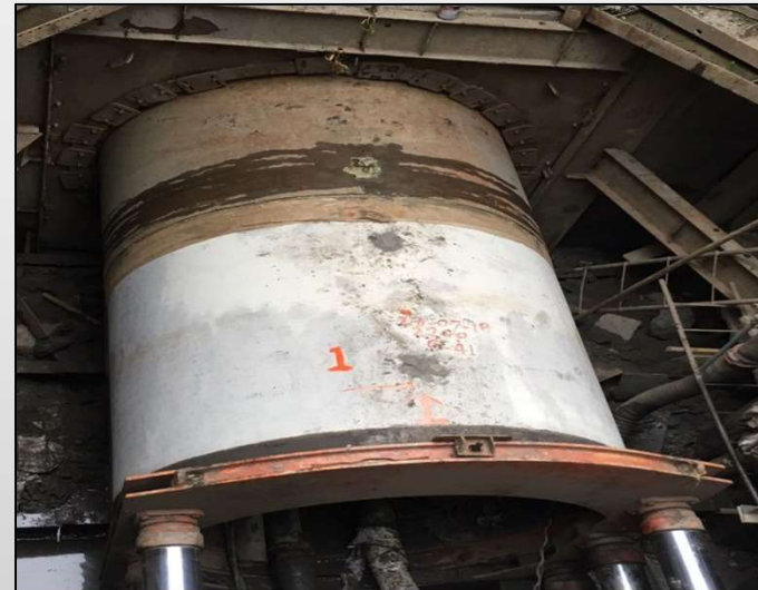
Micro Tunneling at Kolkata
