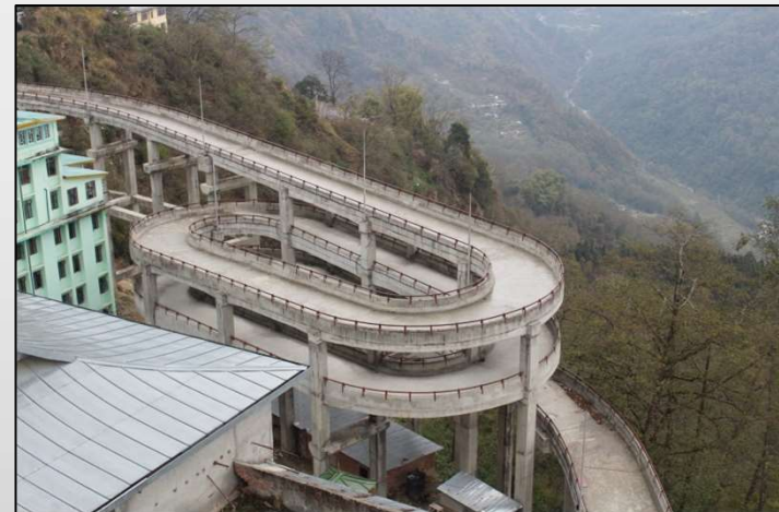
Piling & Civil Works for Gangtok Project
