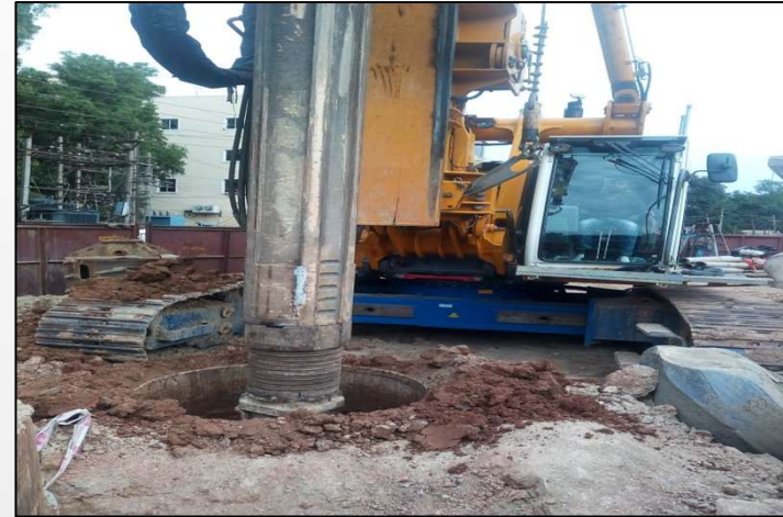
Bangalore Metro Piling Work
