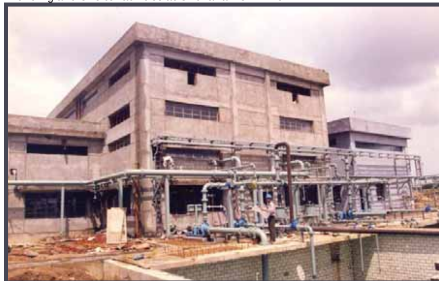
Brakreswar plant building for water supply package
