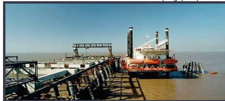
Chemical handling jetty for Gujarat Chemical and Port Terminal
