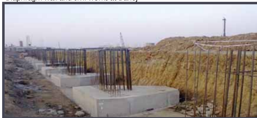
Foundation BASF, Dahej
