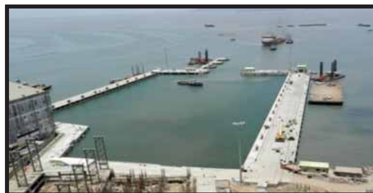
Mazagon Dock Limited
