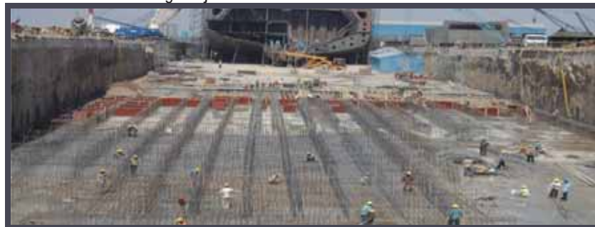
Diaphragm wall and civil works at Dahej
