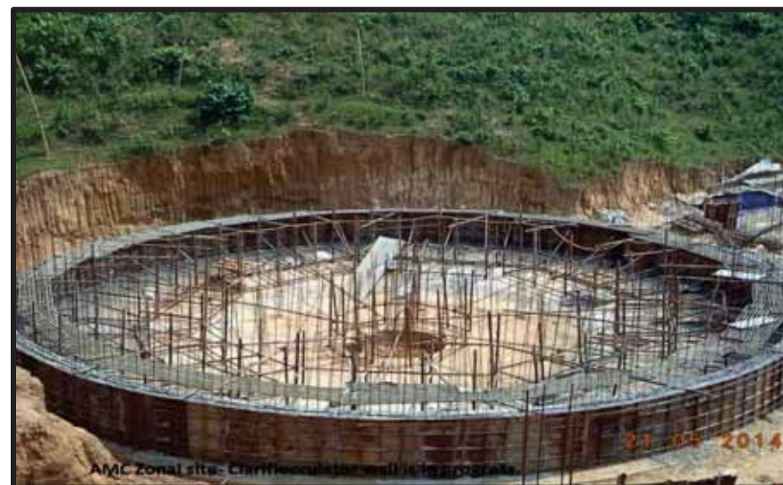
Clariflocculator Wall at Agartala
