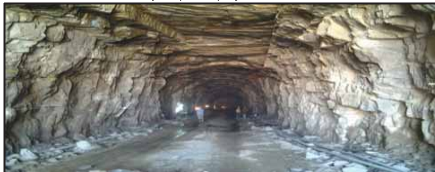
Pranahita - Adit Tunnel-Hard Rock Excavation Completed Stretch
