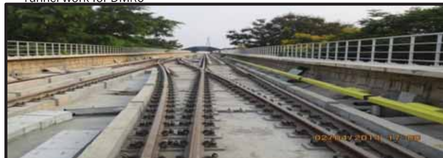
Bangalore Metro Rail Project
