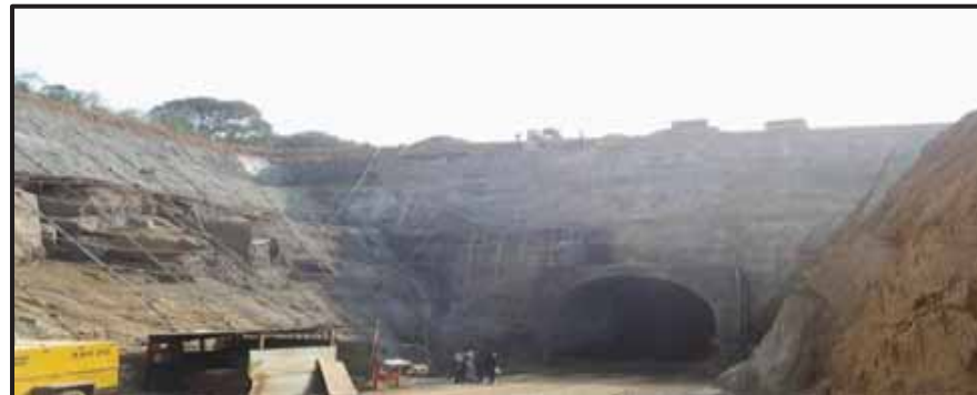
Pranahita - Adit Tunnel Entry Point
