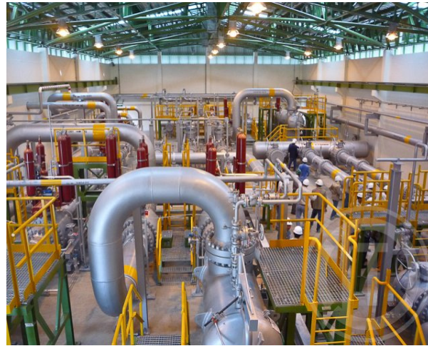
North Bangkok Power Plant Gas Pipeline Project
