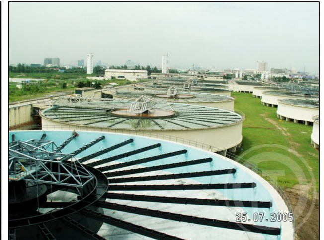
Bang Khen Water Treatment Plant, Bangkok
