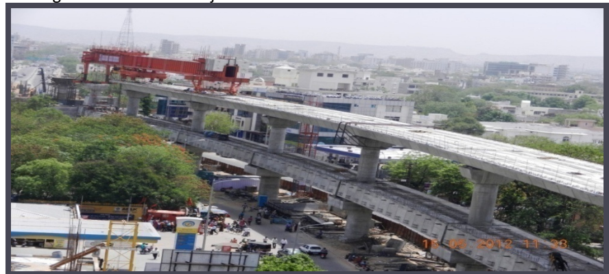
Jaipur Metro Rail Project
