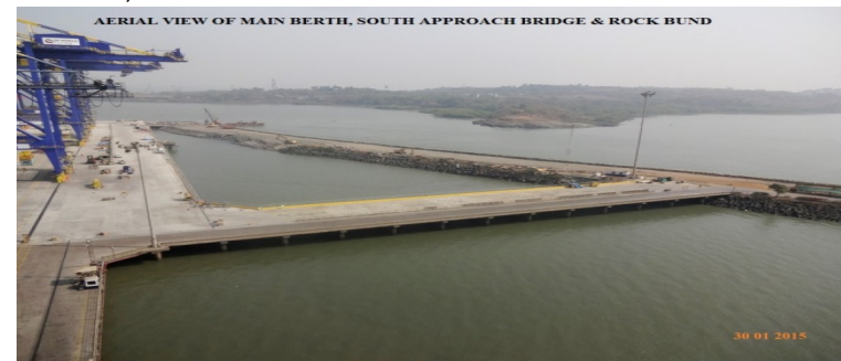
DP World Jetty, Navi Mumbai
