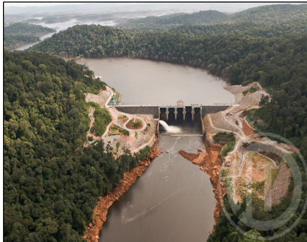
Nam Theun 2 Hydroelectric Project Contract, Laos
