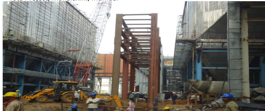
Sasan – Pipe Race work
