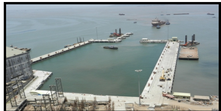
Mazagon Dock Limited
