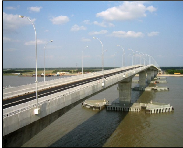
Rupsa Bridge Construction Project, Khulna Bangladesh
