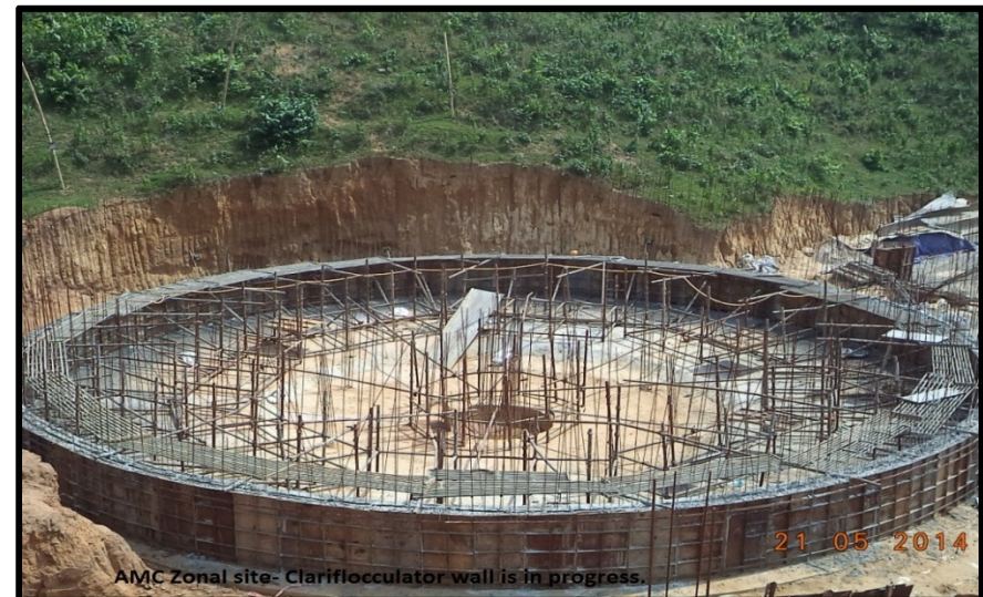
Clariflocculator Wall at Agartala
