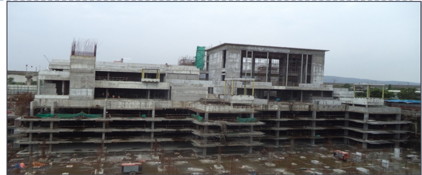
Civil Works Wadala
