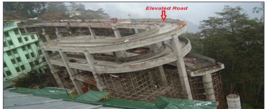
Piling & Civil Arctech, Gangtok
