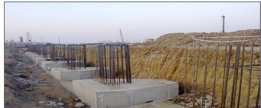
Foundation BASF, Dahej
