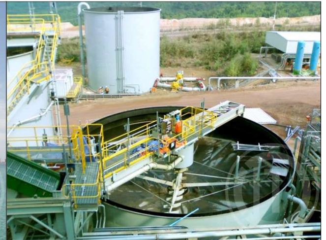
HDPE Tailing and Decant Piping Installation
