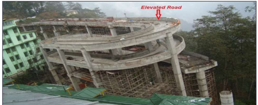
Piling & Civil Arctech, Gangtok
