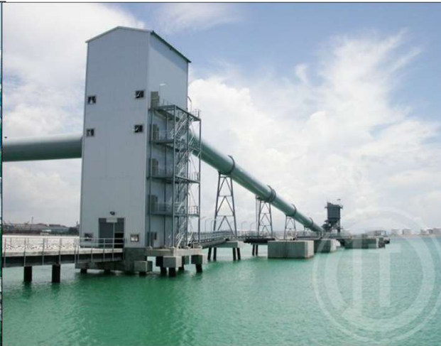
COCO Coal Handling System
