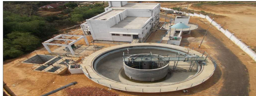
Agartala WTP project
