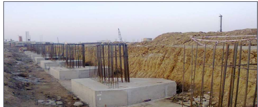
Foundation BASF, Dahej
