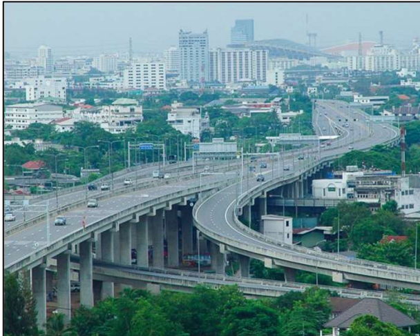
Ramindra - At Narong Expressway System
