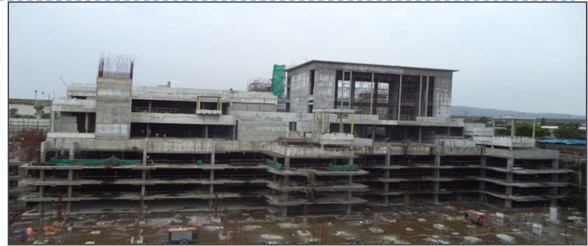
Civil Works Wadala
