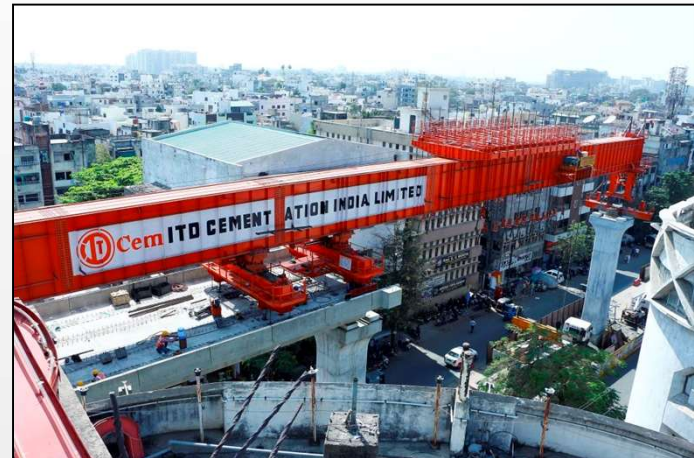
Nagpur Metro Elevated Project
