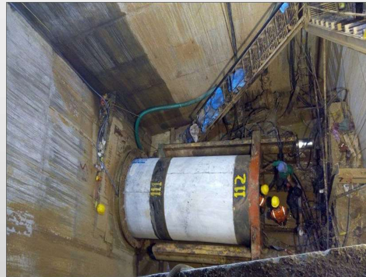
VMSS – Micro Tunneling Vadodara
