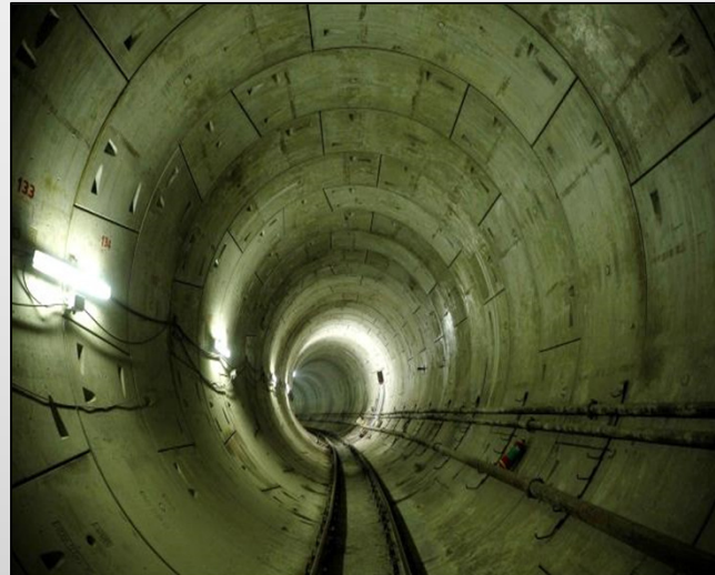
TBM Tunnel
