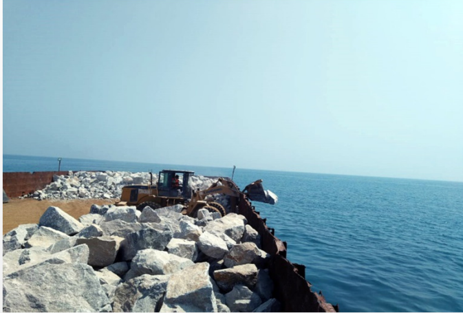
Rock Placing, Udangudi Project
