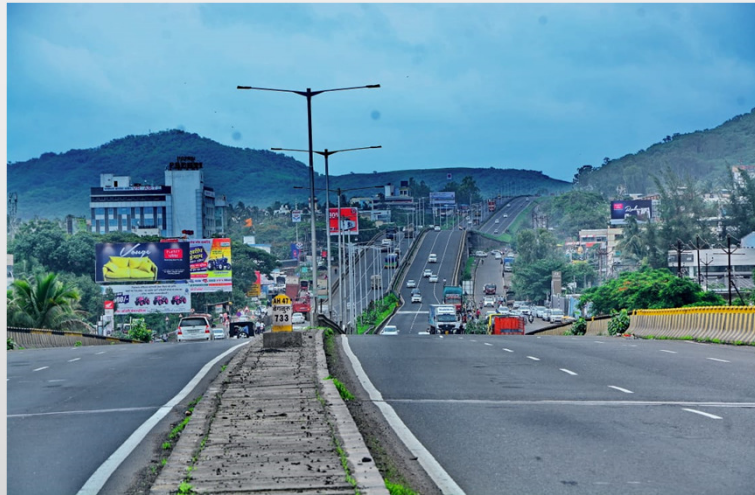
Pune Satara Road Project
