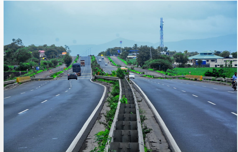
Pune Satara Road Project
