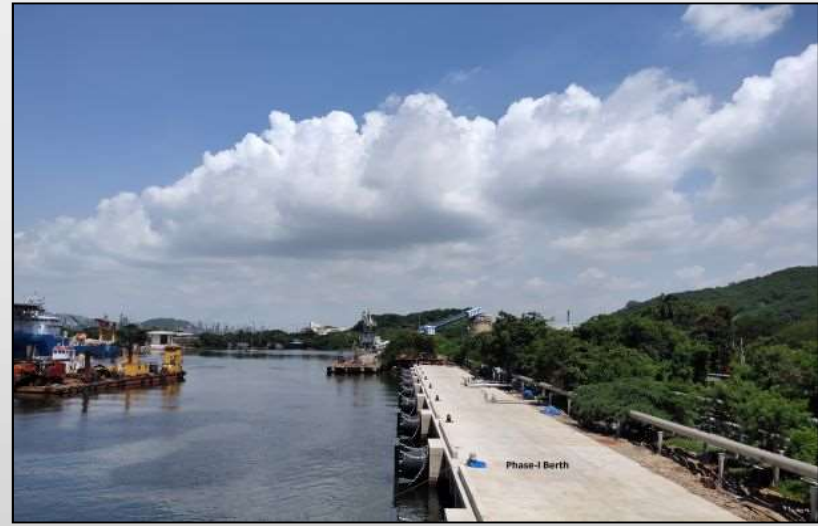
Vizag Port Marine Jetty
