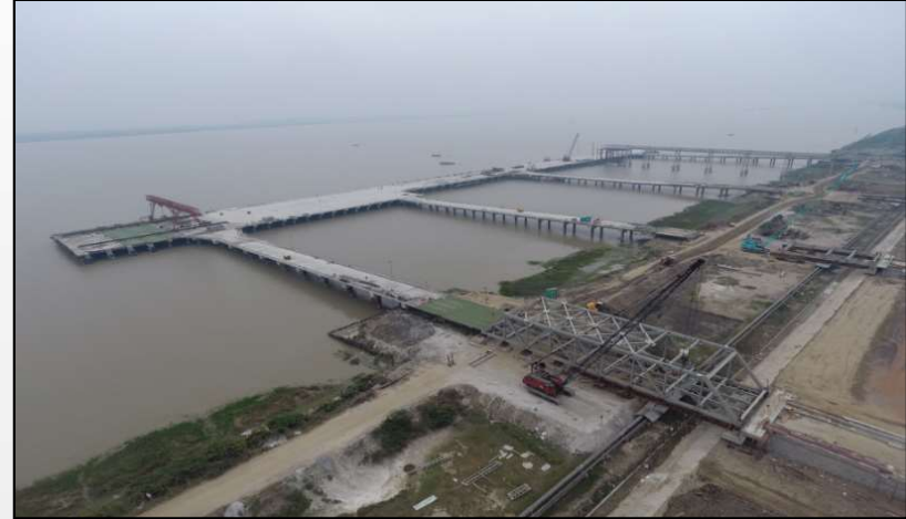
Haldia Inland Waterways Jetty
