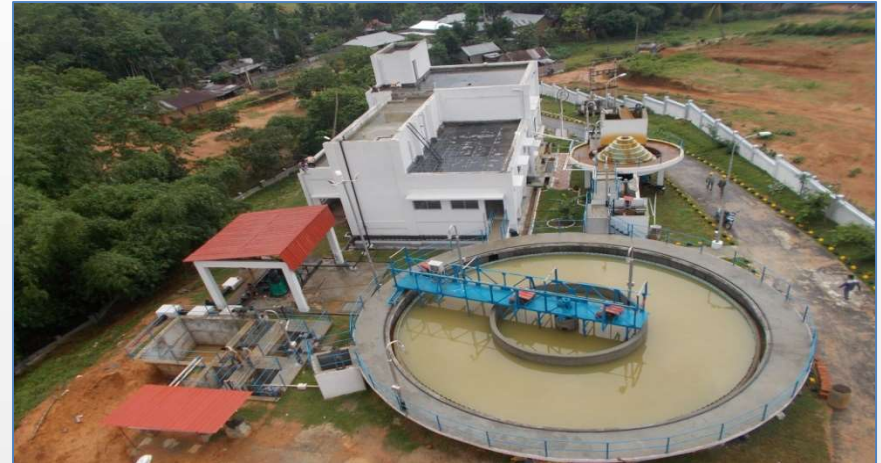
Agartala WTP project
