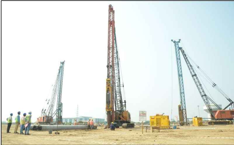
Dahej Spun Pile Project
