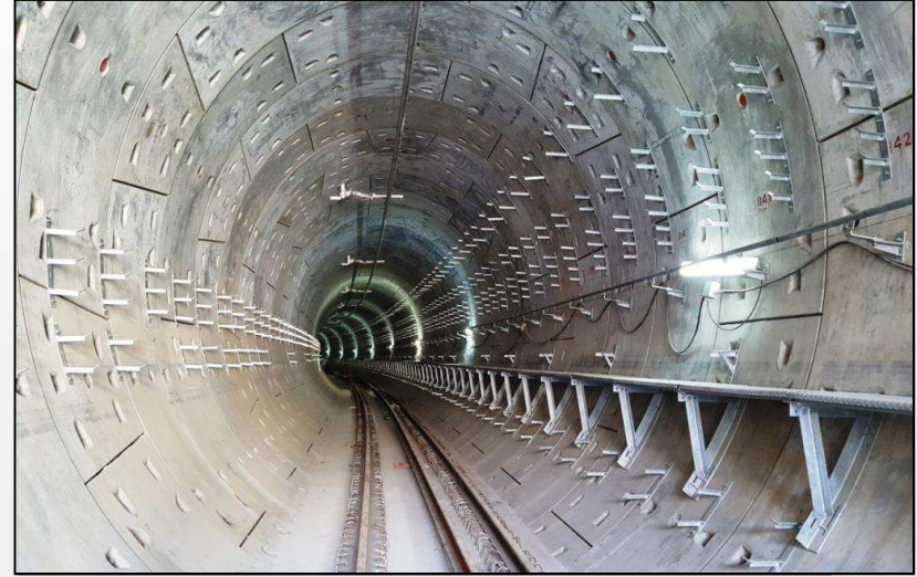
Mumbai Metro Underground Tunneling Project
