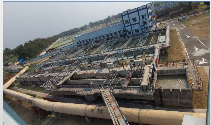
Palta WTP, West Bengal
