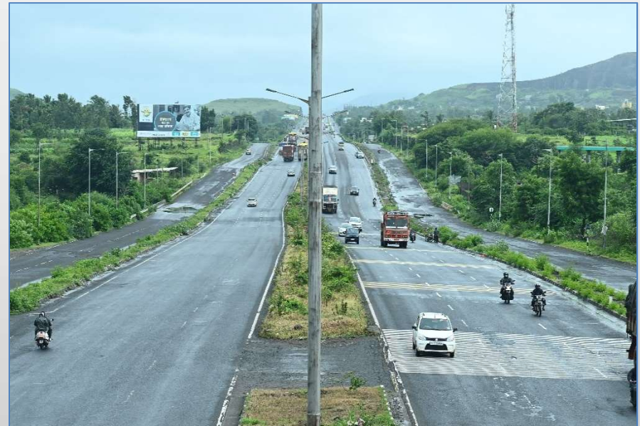
Pune Satara Road Project
