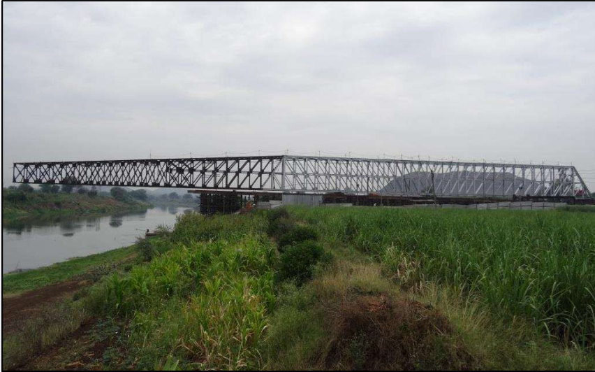
Dharna Bridge, Nashik
