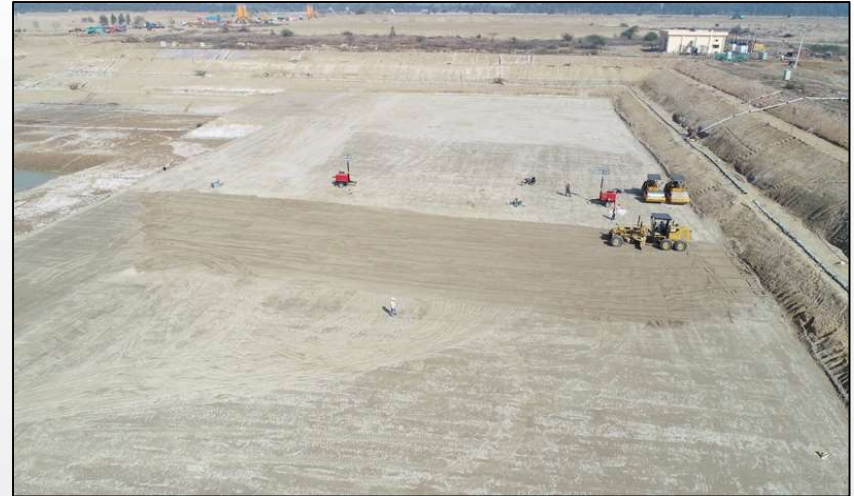
Ground Stabilization work, Haryana
