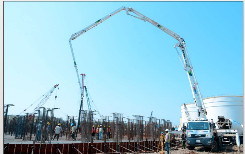
Precast Piling Project, Kandla
