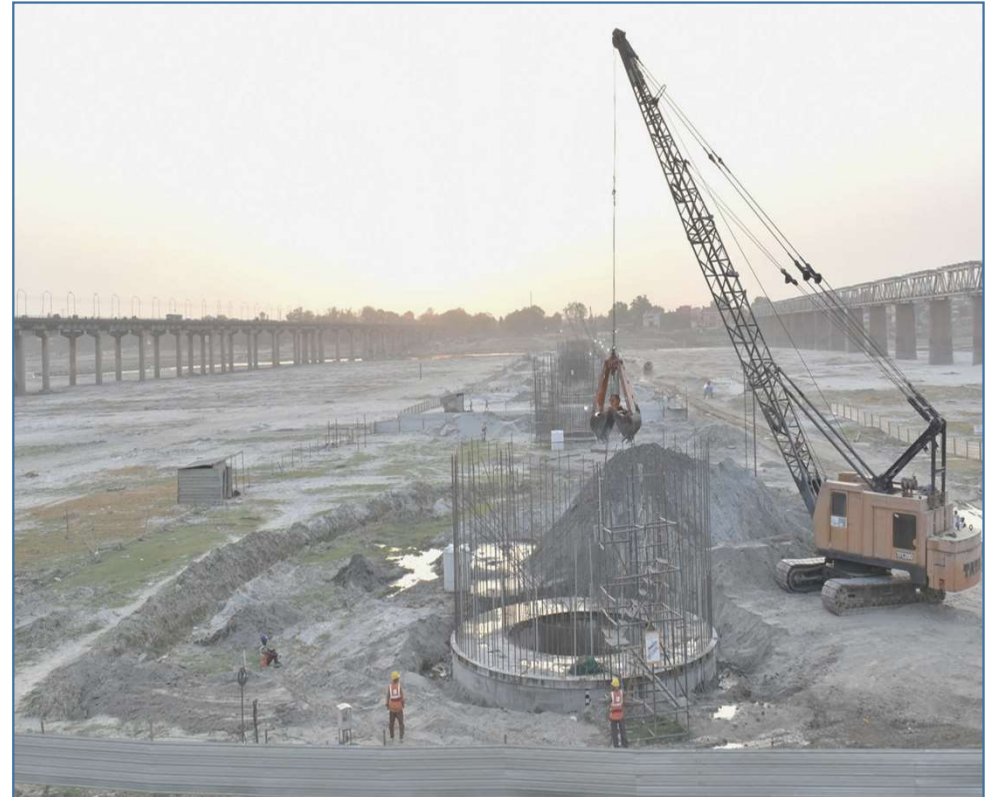
Ganga Steel Bridge project in Uttar Pradesh
