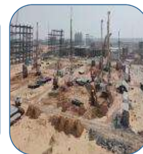
FOUNDATION AND SPECIALIST ENGINEERING
