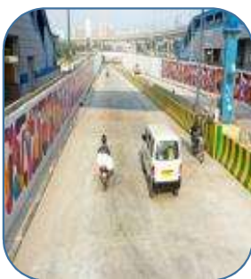
HIGHWAYS, BRIDGES AND FLYOVERS
