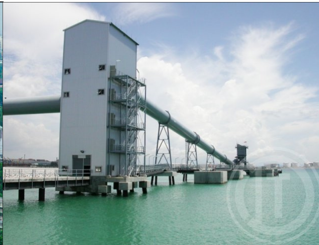
COCO Coal Handling System
