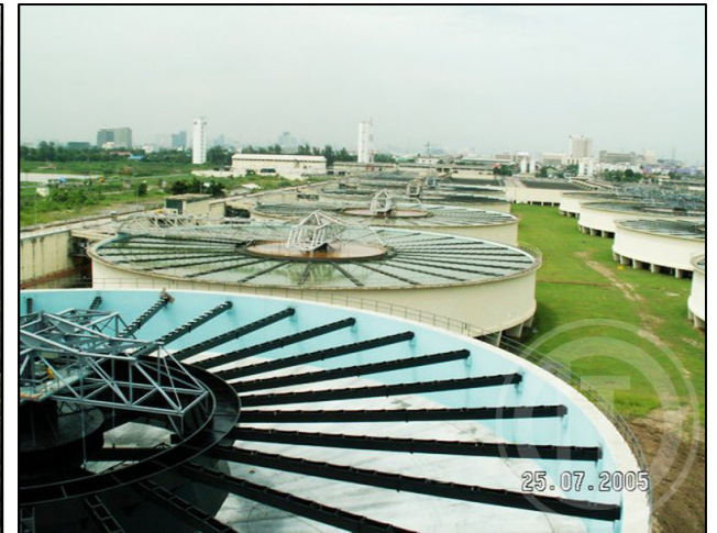
Bang Khen Water Treatment Plant , Bangkok
