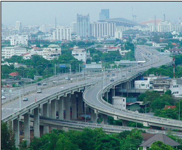
Ramindra - At Narong Expressway System
