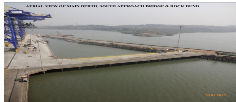
DP World Jetty, Navi Mumbai
