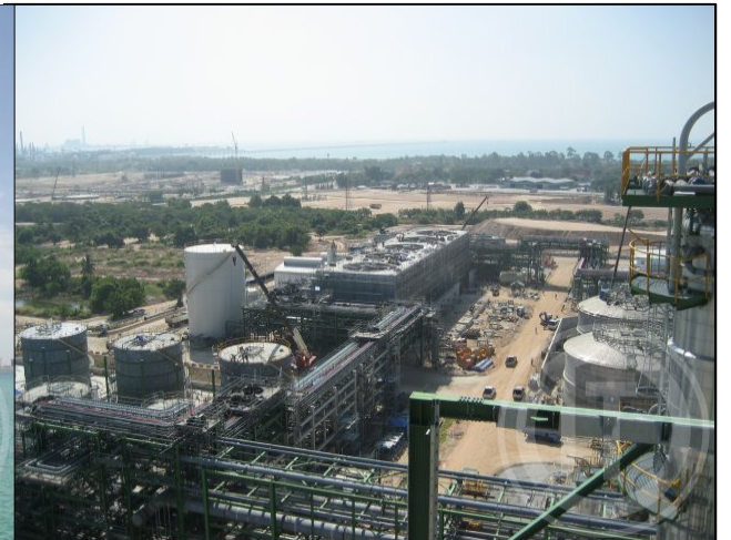
Piping works for PTT phenol project
