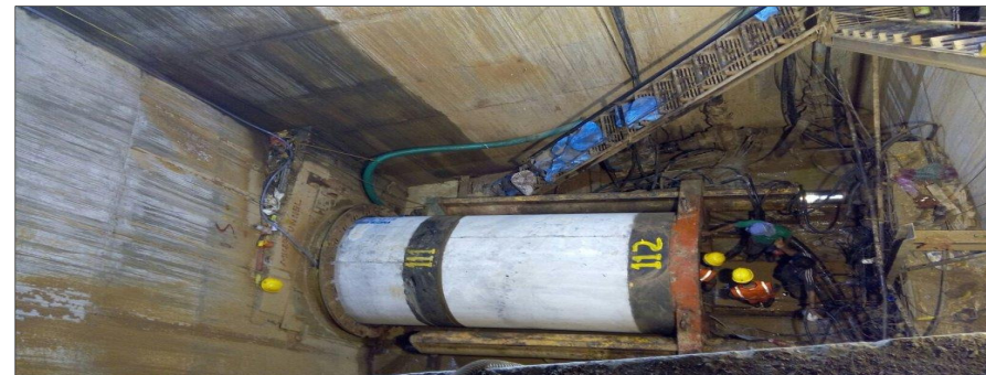
VMSS – Micro Tunneling Vadodara
