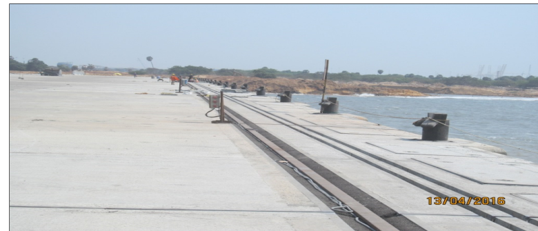
Ennore container terminal, Chennai
