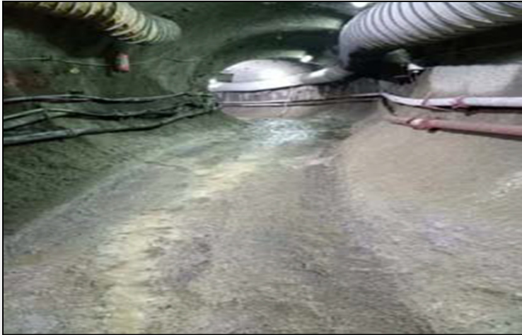
Underground Kolkata Metro Project
