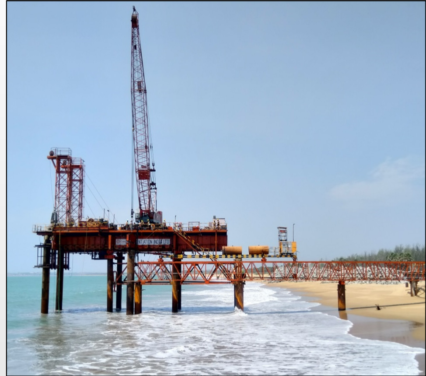
Udangudi, Tamilnadu Power Project
