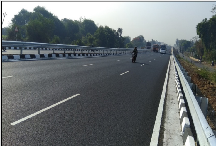
Pune Satara Road Project
