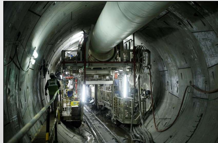
TBM Tunnel, Mumbai Metro
