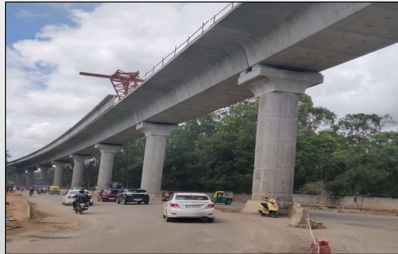
Bangalore Metro – In Progress
