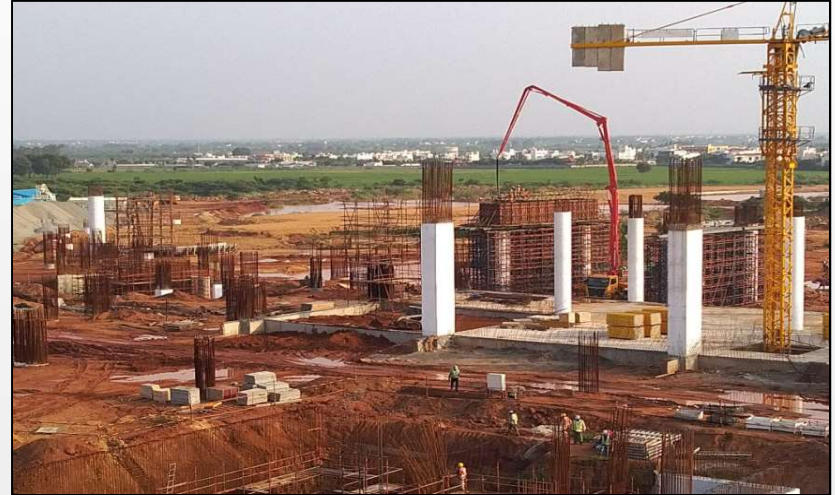
Trichy Airport Modernization - In Progress
