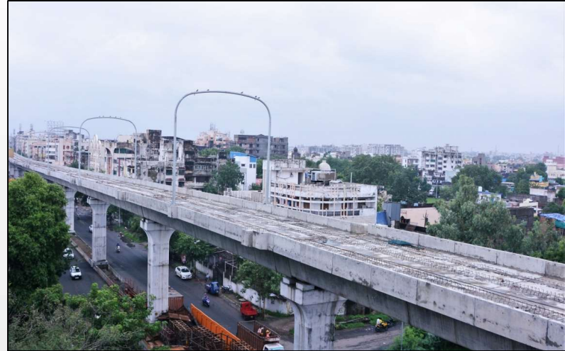
Nagpur Metro Viaduct
