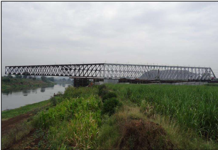
Dharna Bridge, Nashik
