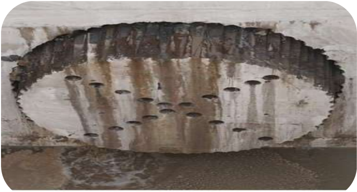
MCGM micro tunnel breakthrough in Mumbai
