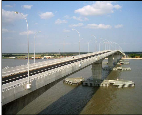
Rupsa Bridge Construction Project, Khulna Bangladesh
