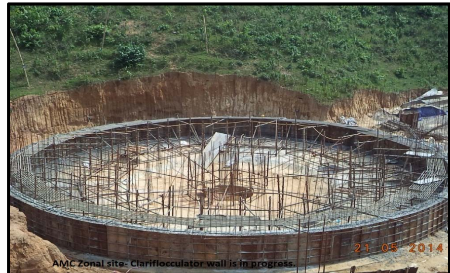
Clariflocculator Wall at Agartala
