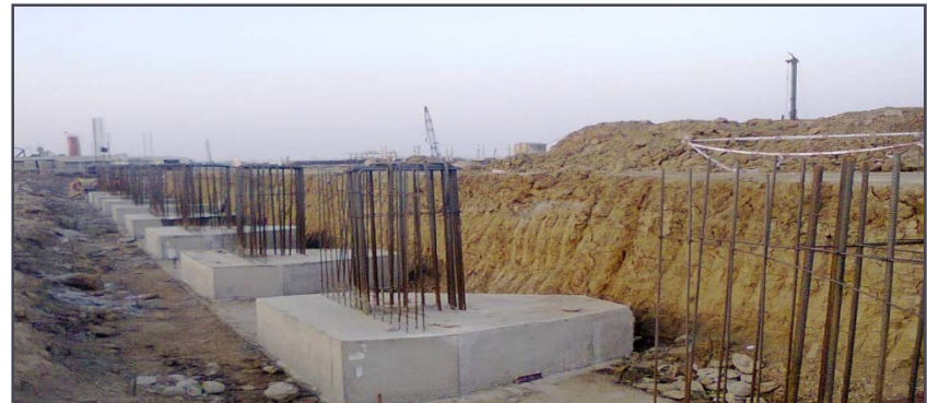
Foundation BASF, Dahej
