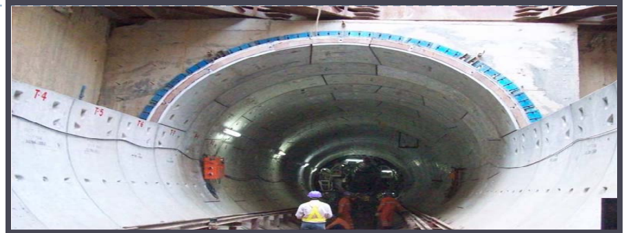
Tunnel work for DMRC
