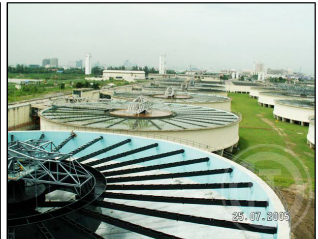
Bang Khen Water Treatment Plant, Bangkok
