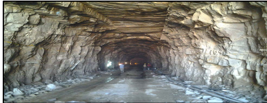
Pranahita - Adit Tunnel-Hard Rock Excavation Completed Stretch
