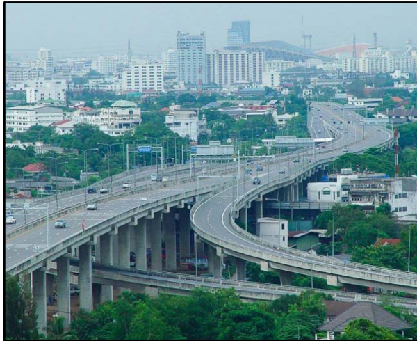
Ramindra - At Narong Expressway System
