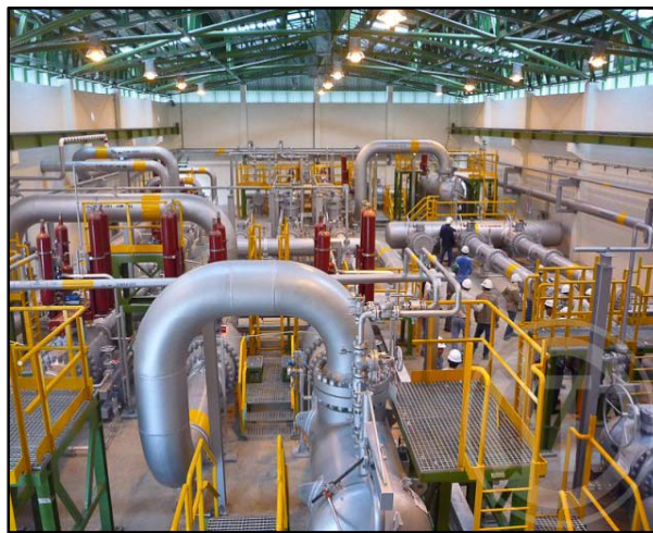
North Bangkok Power Plant Gas Pipeline Project
