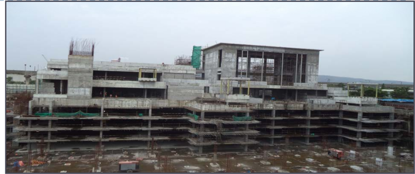
Civil Works Wadala
