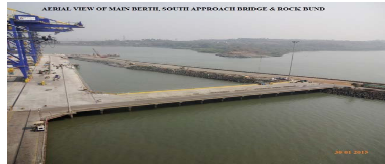
DP World Jetty, Navi Mumbai
