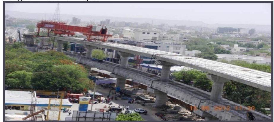
Jaipur Metro Rail Project
