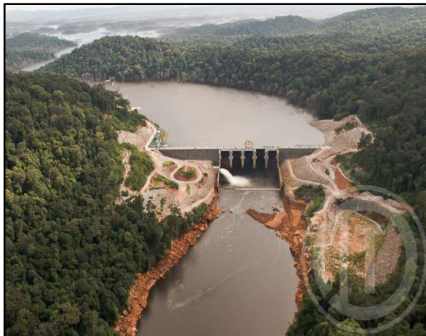
Nam Theun 2 Hydroelectric Project Contract, Laos
