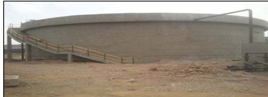
Kawai Project – Sludge Thickener
