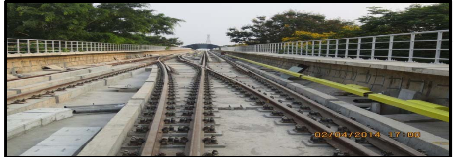
Bangalore Metro Rail Project
